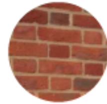
Lower Walls - Brickwork
