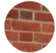
Lower Walls - Brick
