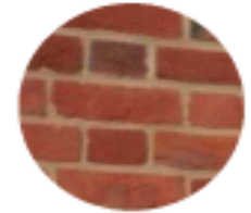
Lower Walls - Brick
