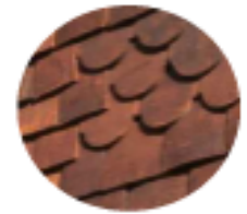
Upper Walls - Tile hanging
