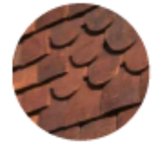
Upper Walls - Tile hanging
