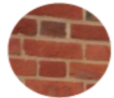
Lower Walls - Brick
